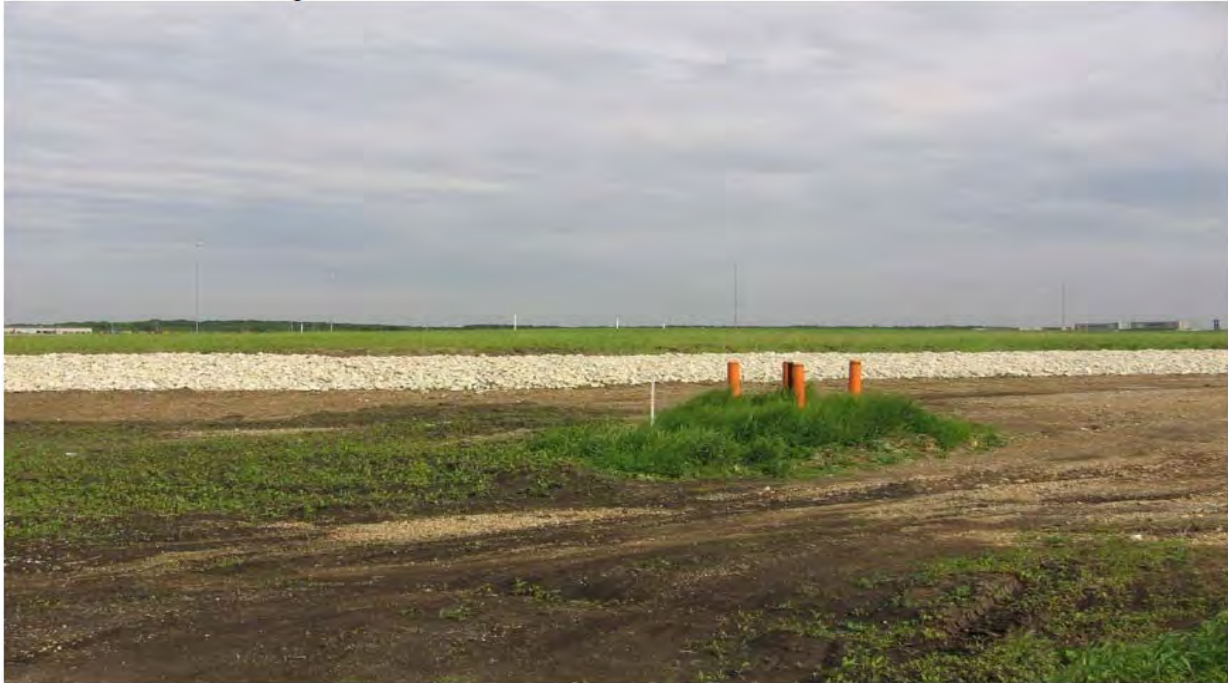
Completed M13 Cap looking SE from NW corner, August 2008
