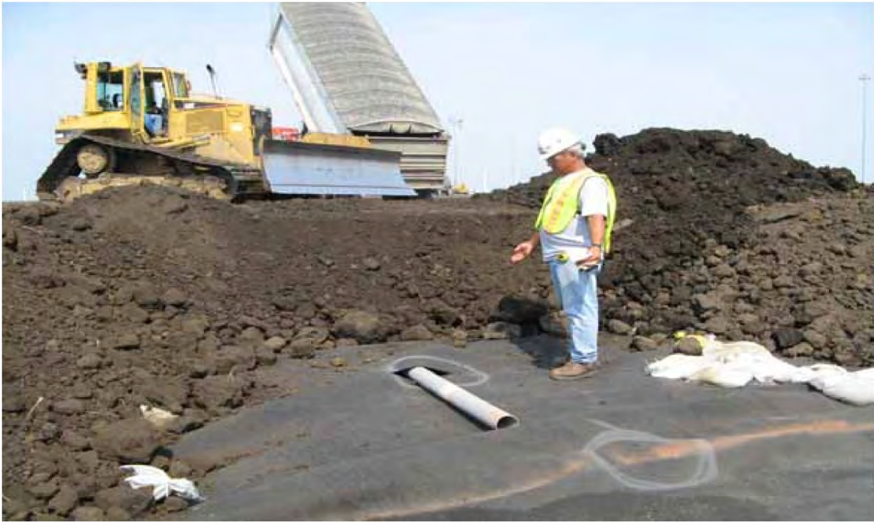
M13 Cap Construction showing the geocomposite membrane, rooting zone, and vent installation.
