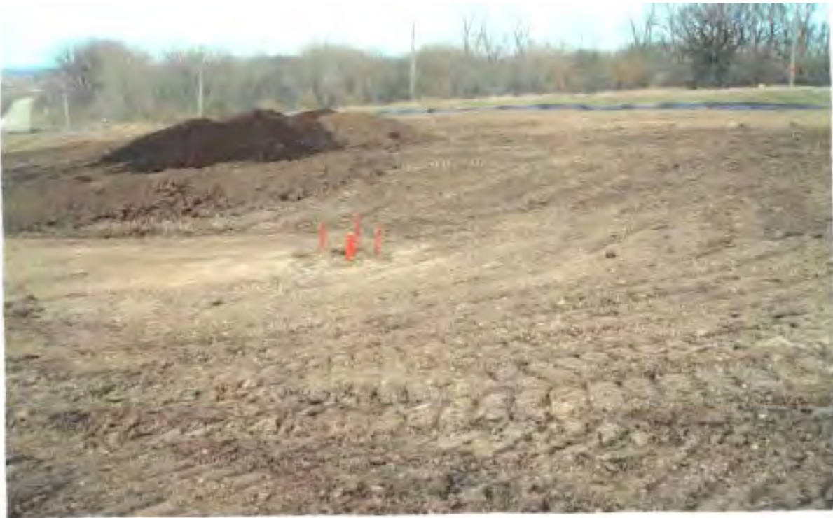
Placing the vegetative layer (treated soils)
